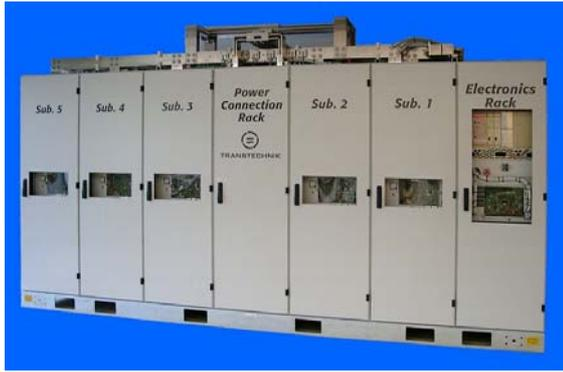
Figure 9. [13kA, 18V] converter
