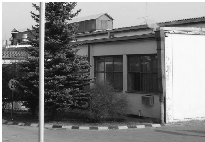
Fig. 7: Thermovision/photo record of a building with losses in vapour distribution.
