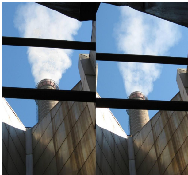
Fig. 14. The left part of the figure illustrates the smoke appearance in configuration of 4 x 50 Hz. The right part of the figure illustrates the smoke appearance in configuration of 2 x 50 Hz + 2 x HF.
