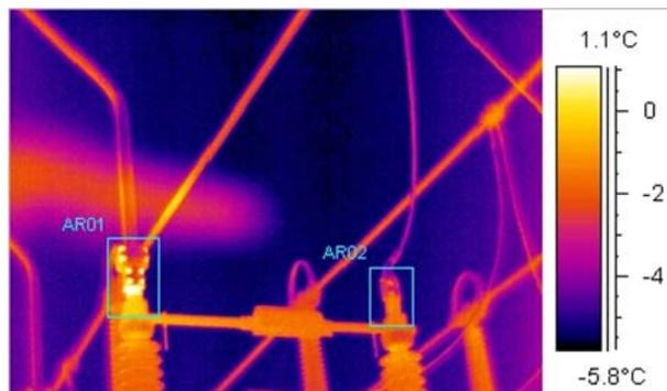
Figure 7. Disconnector F0 in TL 110 kV Višegrad in the FU 110/20/10 kV Goražde 2
